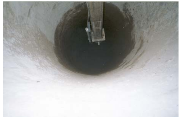
Lowering the Kelly bar past the upper casing
