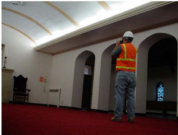
Videotaping an Existing Structure
