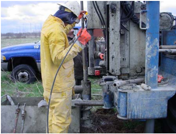
Feeding the pressuremeter into the borehole
